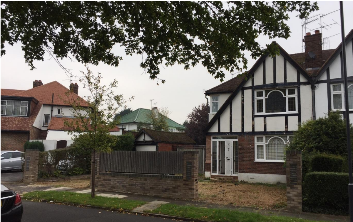
Front elevation of the application site
