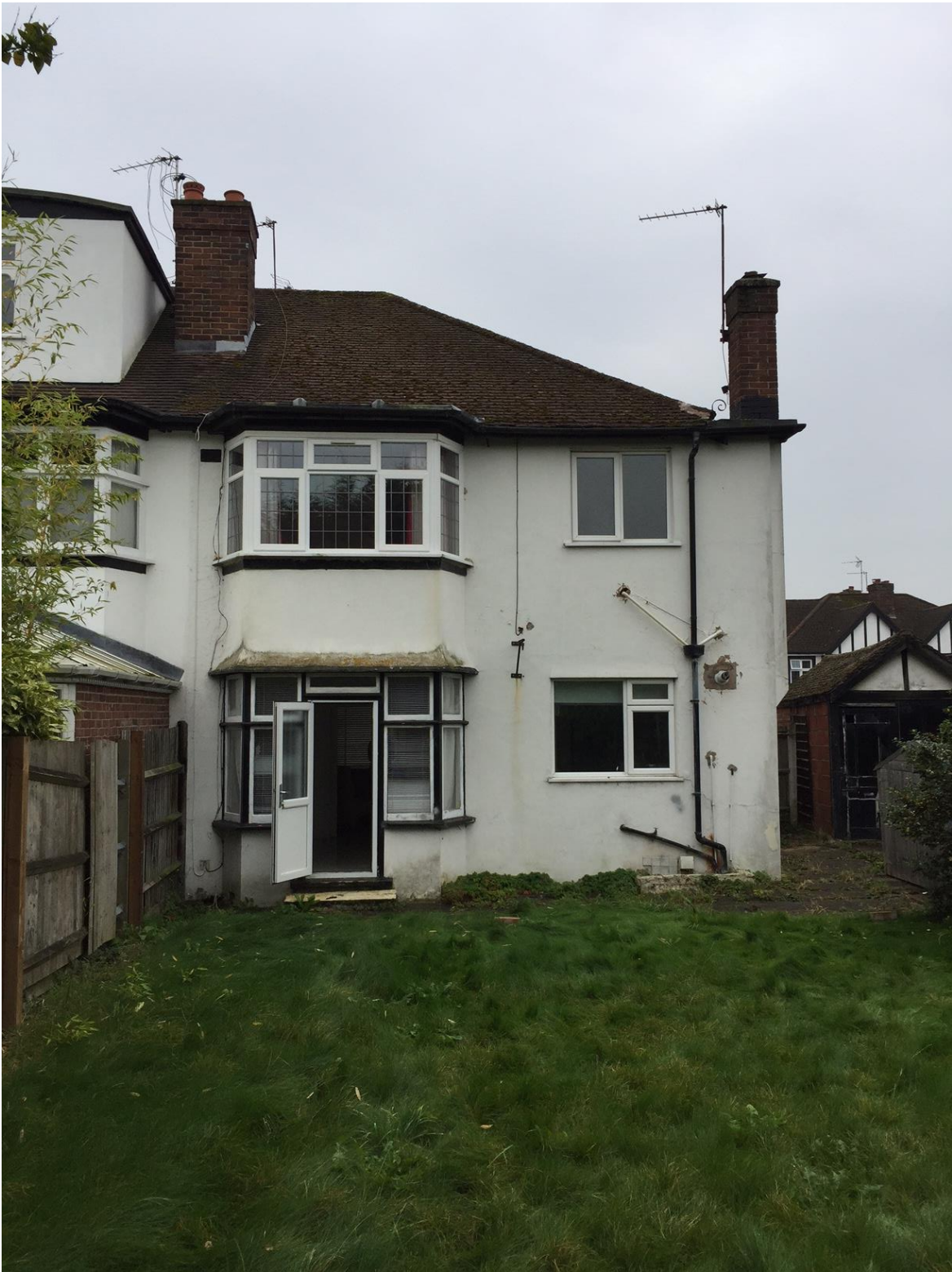
Rear elevation of 11 Sherington Avenue
