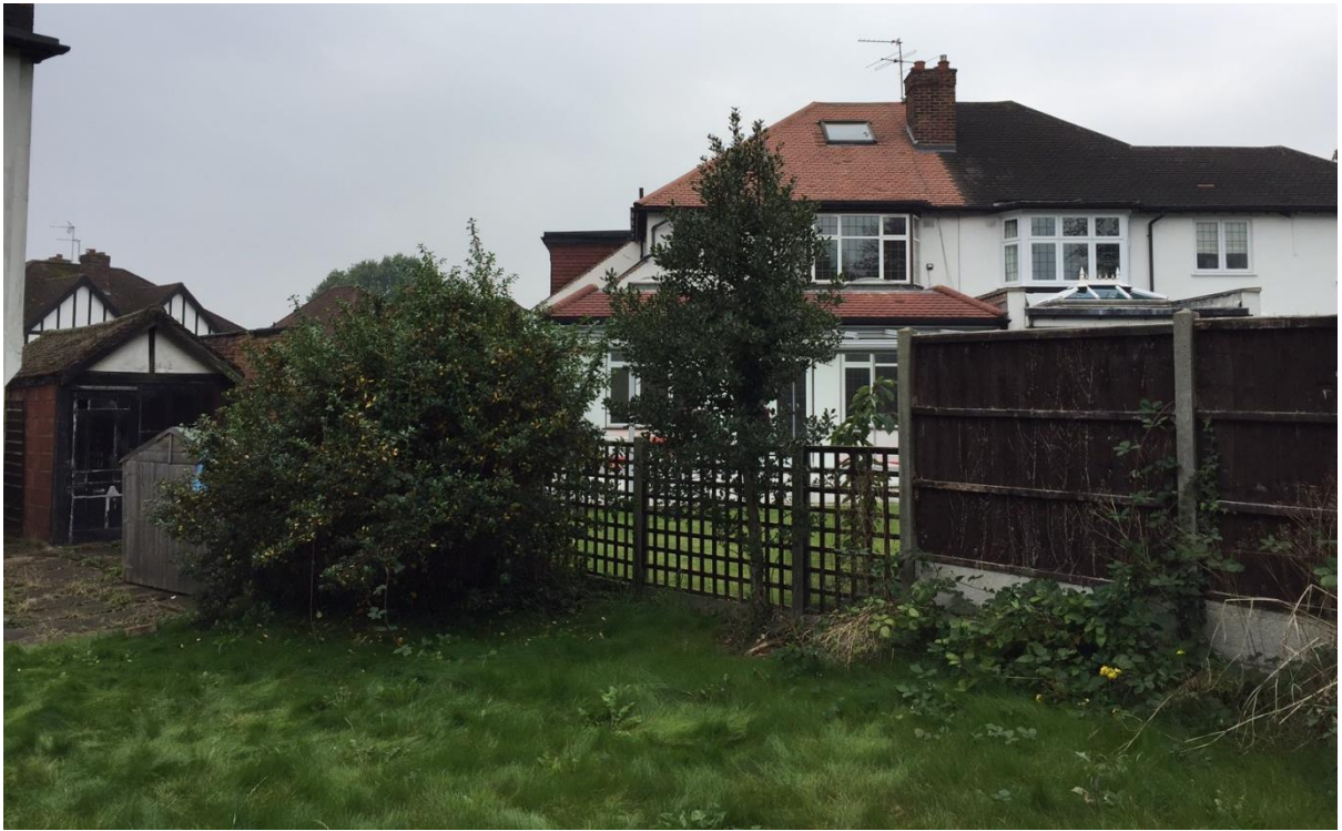
Rear elevation of neighbouring properties No.9 Sherington Avenue and the adjoining property No.2 Furham Feild
